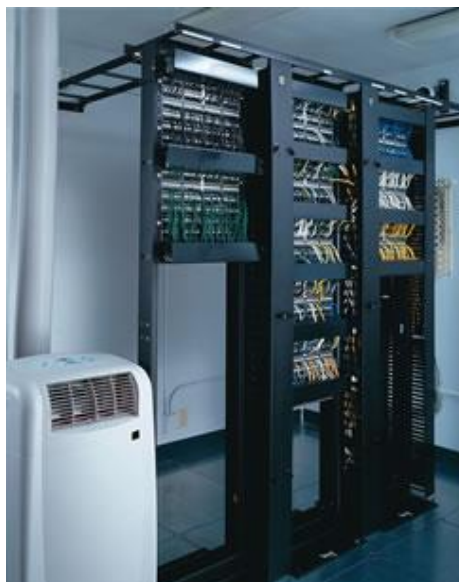
Rural Microgrids and Telecoms
